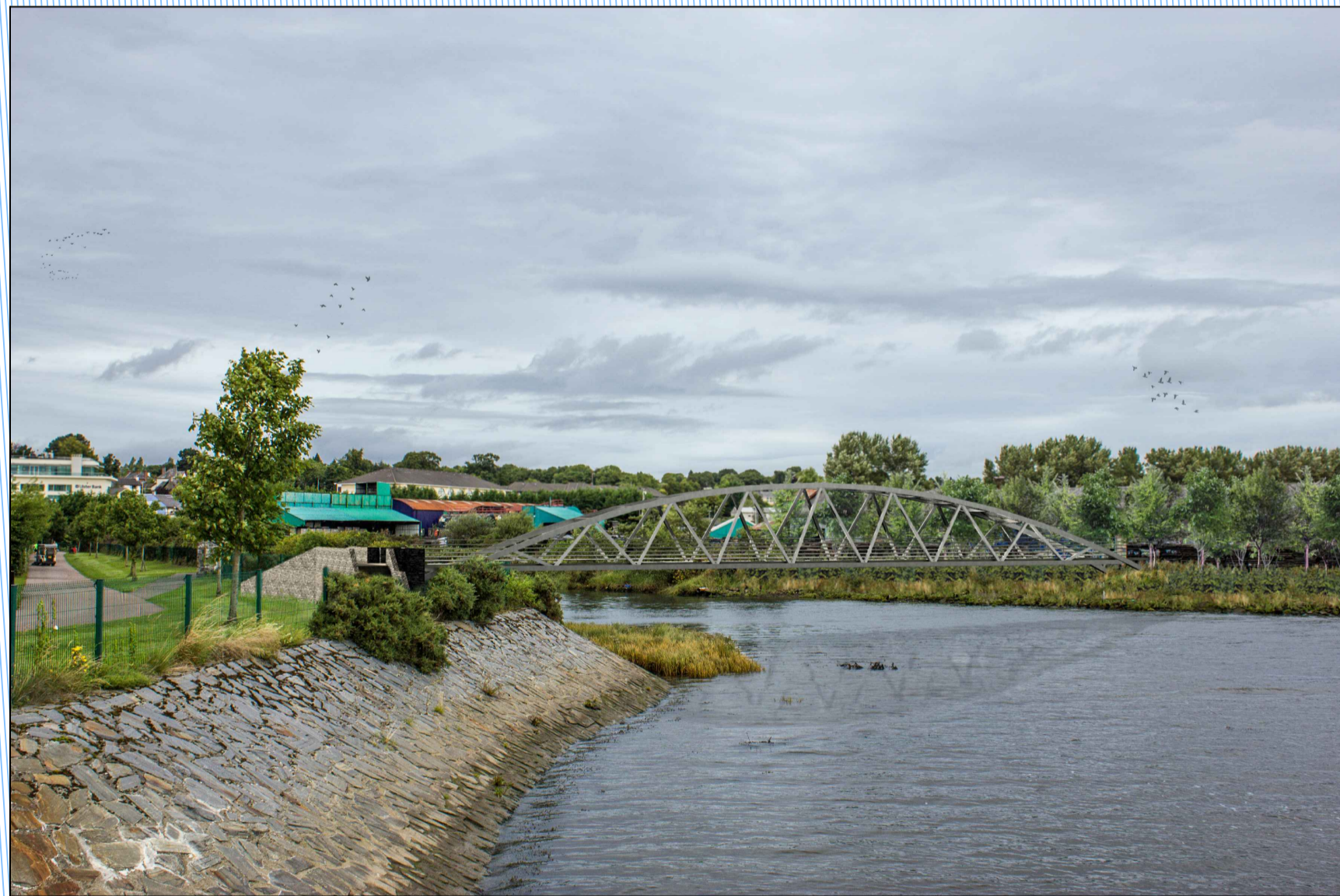
Visual 1 - Bay Road Bridge (B)
